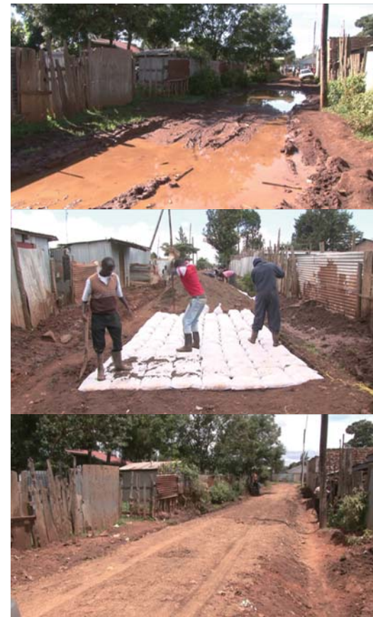
Road improvement using Kimura's method
